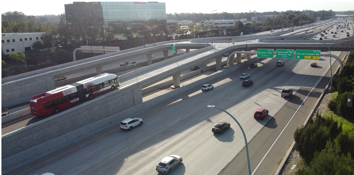
Image: I-15 Mira Mesa Direct Access Ramp to San Diego Miramar College Transit Station
