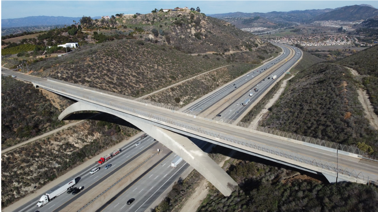
Image: Lilac Road Bridge over I-15 in San Diego County..
