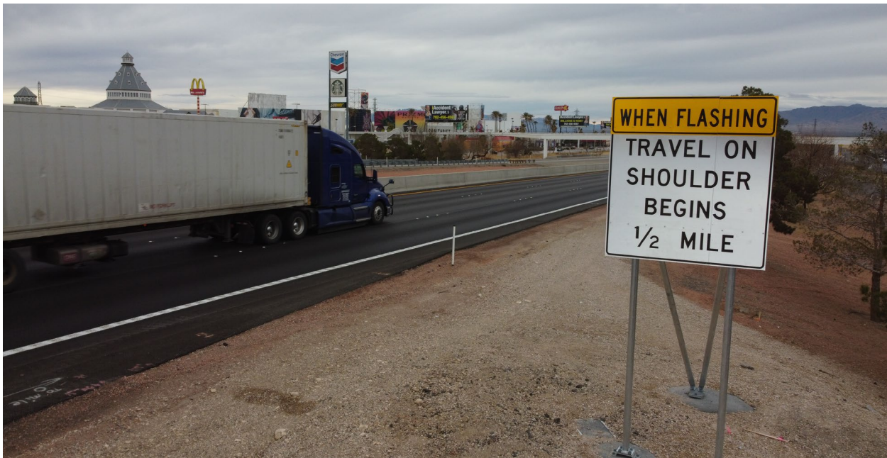
Image: a joint California and Nevada pilot project on I-15 southbound from Primm, NV to CA Agriculture Station that utilizes the shoulder into temporary third lane during periods of peak congestion.
