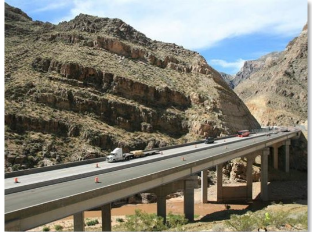
Image: I-15/Virgin River Gorge Bridge (Credit: ADOT)
