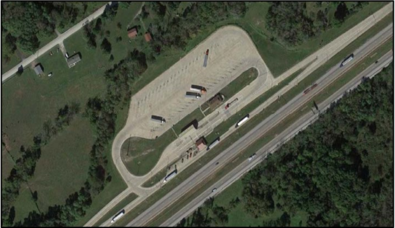
Figure 3-3: Truck Parking at Weigh Station Example
