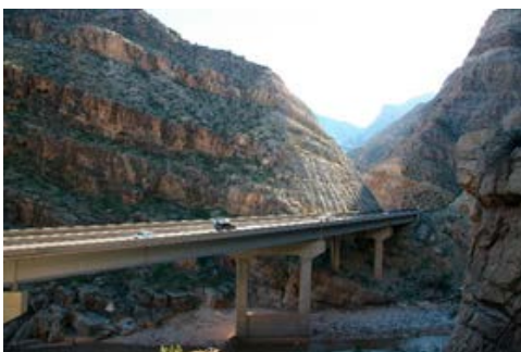
Virgin River Gorge Bridges Reconstruction (Arizona)
