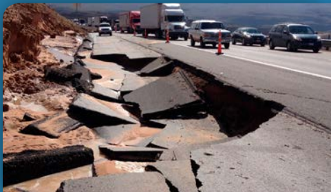
I-15 flood damage, September 2014
