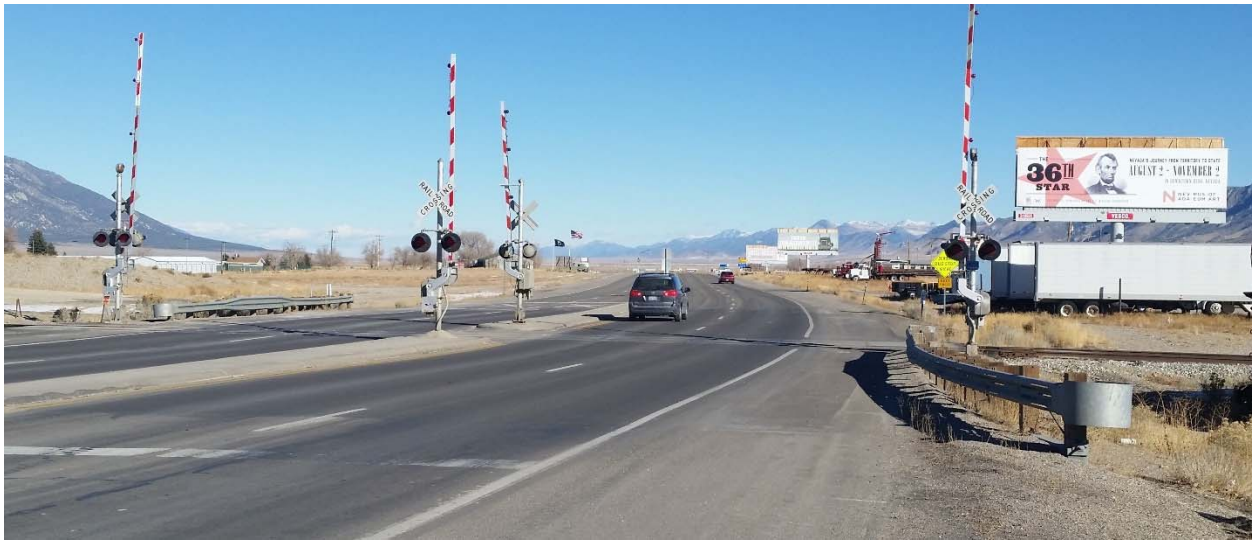
Figure 3-14. Railroad Crossing on US 93 at Ely, Nevada
