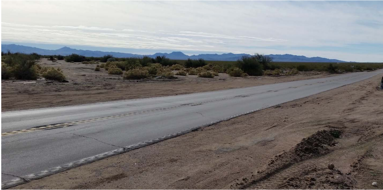
Figure 3-9. No Storm Drains or Culverts on US 95 in California Allow Storm Water to Overtop the Roadway
