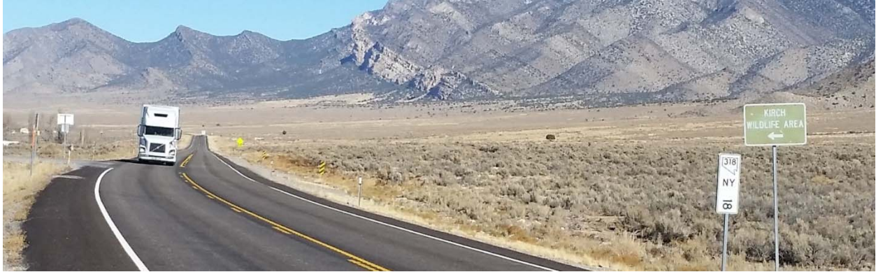
Figure 3-11. No Turn Lanes on NV 318 for the Kirch Wildlife Area
