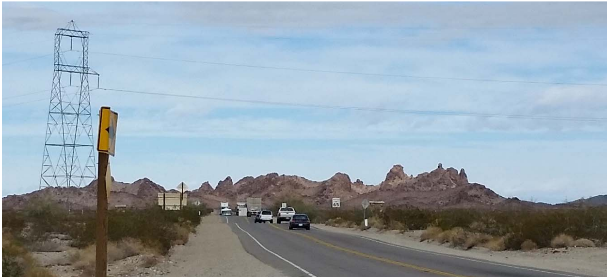
Figure 3-8. US 95 in California has a High Volume of Trucks and RVs, and Few Opportunities for Safe Passing
