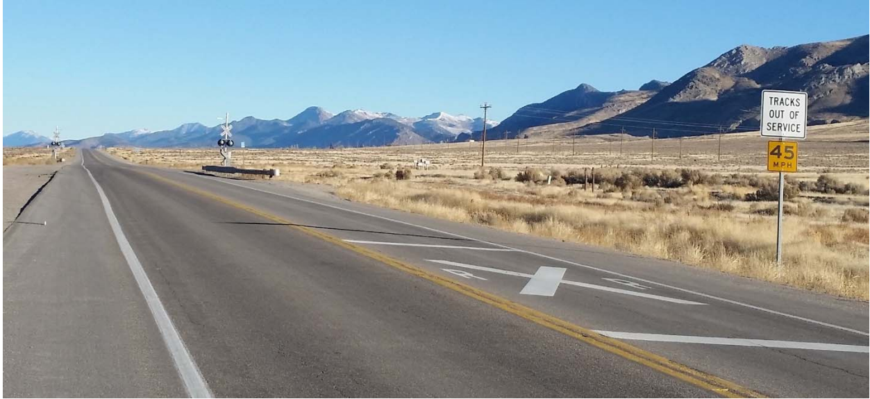
Figure 3-13. Railroad Crossing on US 93 near McGill, Nevada
