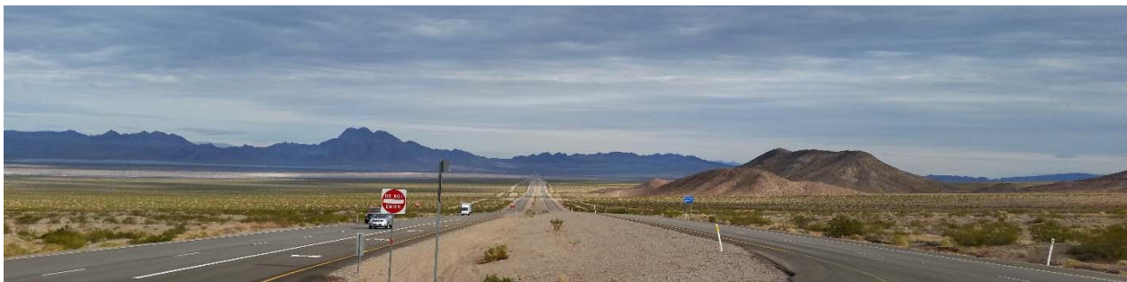
Figure 3-6. US 95 in Nevada is Mostly 4-Lane Divided Highway
