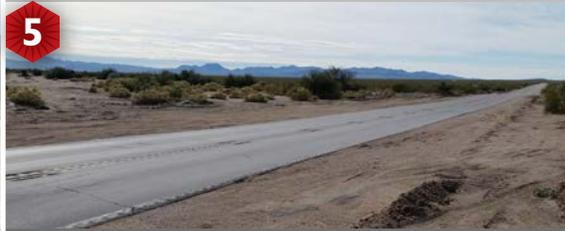
**Constraint:** US 95 in California follows the contour of the surrounding terrain allowing storm water to overtop the roadway. A major wash crosses US 95, frequently closing the highway during major storm events
